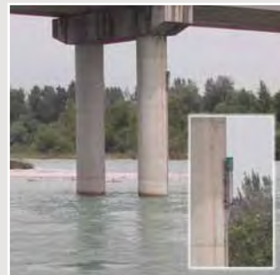
Flood warning installation with self-sufficient solar power supply
